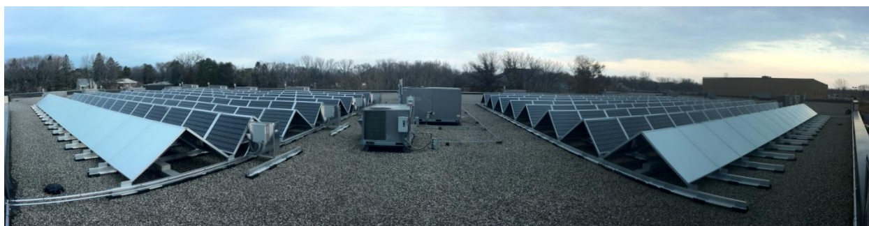
A leased 40-KW solar system on a commercial building roof. The system owner (Solarflow) rather than the building owner (Transfiguration Church), maintains the system.
